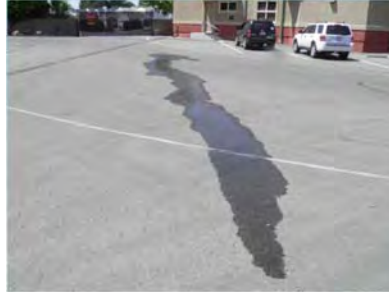
Two gallon spill on sloped surface
