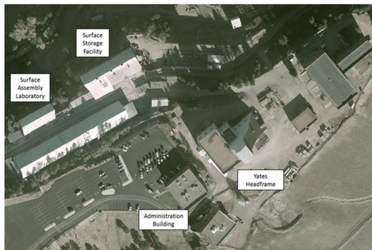
Figure 10.1.1: Aerial view of the SURF site showing the locations of the Surface Assembly Laboratory and the Surface Storage Facility.
