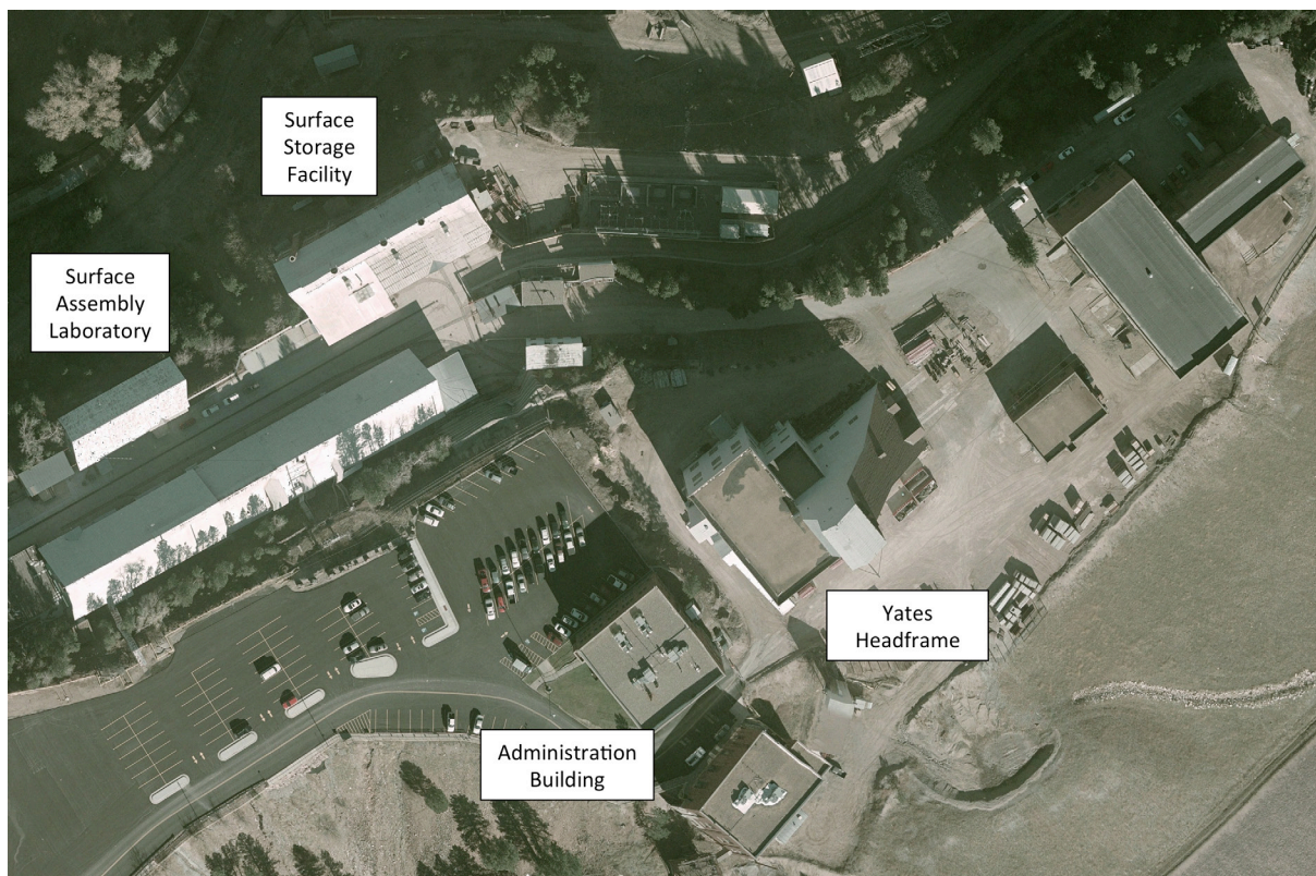
Figure 13.1.1 Aerial view of the SURF site showing the locations of the Surface Assembly Laboratory and the Surface Storage Facility.
